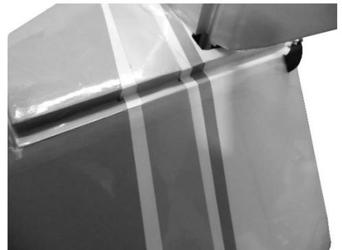
Seal the entire hinge gap while rudder is fully deflected
